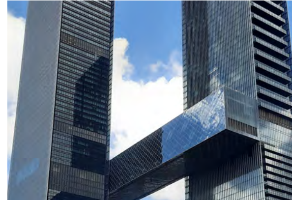
One Zaabeel Tower- Apartment
